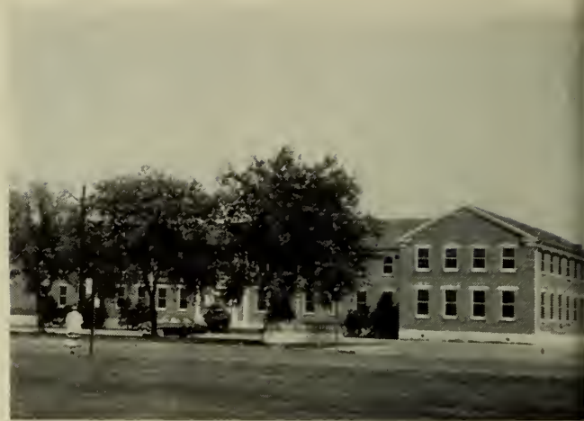
Headquarters building of Air Finance Center, Denver, new home of the Continental Air Command's Air Reserve Records Center.
