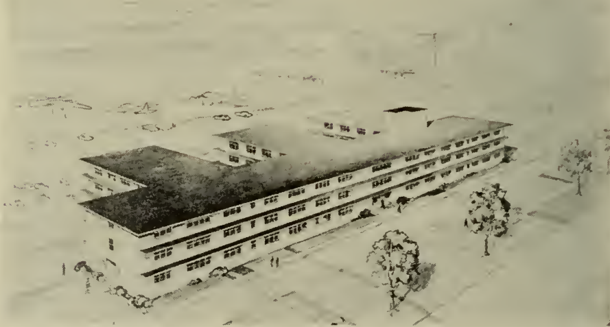
Site preparation is underway at Robins AFB, Ga, on this $897,600 headquarters building for Fourteenth Air Force. The building will have a floor area of approximately 90,000 square feet and be of concrete block construction. The architect's drawing above shows the building which will be used to house records and personnel of Hq Fourteenth Air Force to serve about 60,000 Air Force Reservists in 12 southern states.
